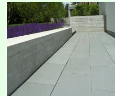
In situ concrete steps and seating edge
